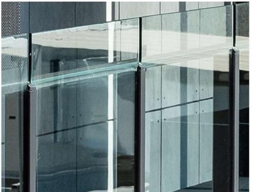
AMW01 - ALUMINIUM FRAME WINDOW & BALUSTRADE SYSTEM
